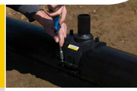
For the simple creation of branches on PE pipes AGRU spigot saddle was developed. The spigot saddle is made of premium PE 100-RC and guarantees a simple installation and absolute reliability. With a spigot saddle, creating a branch on existing pipe has become much simpler and cost-effective.
